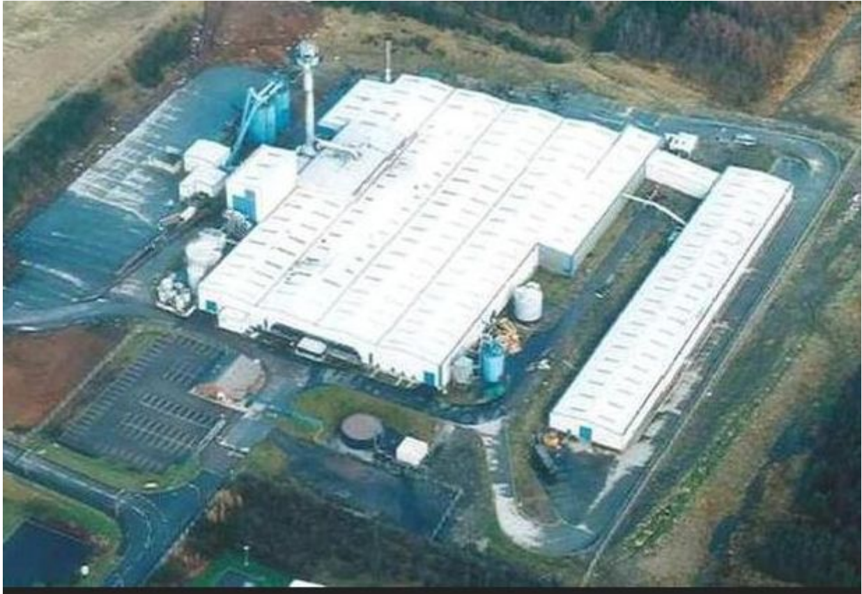
TVR factory aerial view.
