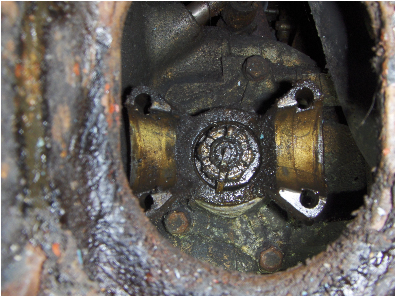
Differential driving flange as first viewed through the drive shaft subframe hole.
