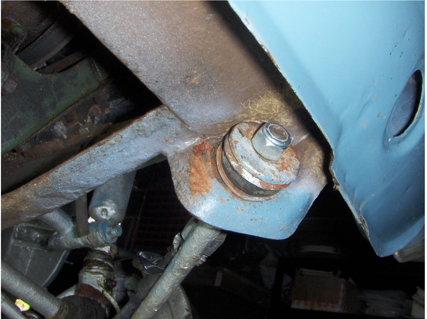
New nut and bushes sited at forward end of tie rod. Not as rusty as it looks (honest!).
