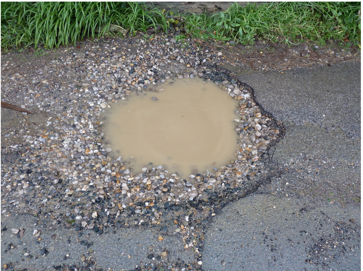
Potholes – Enemies of car wheels, tyres and suspension systems. Photograph © Kim Henson.
