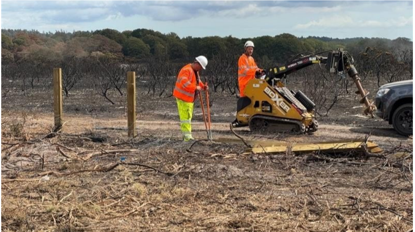
A31 boundary fence replacement work.
