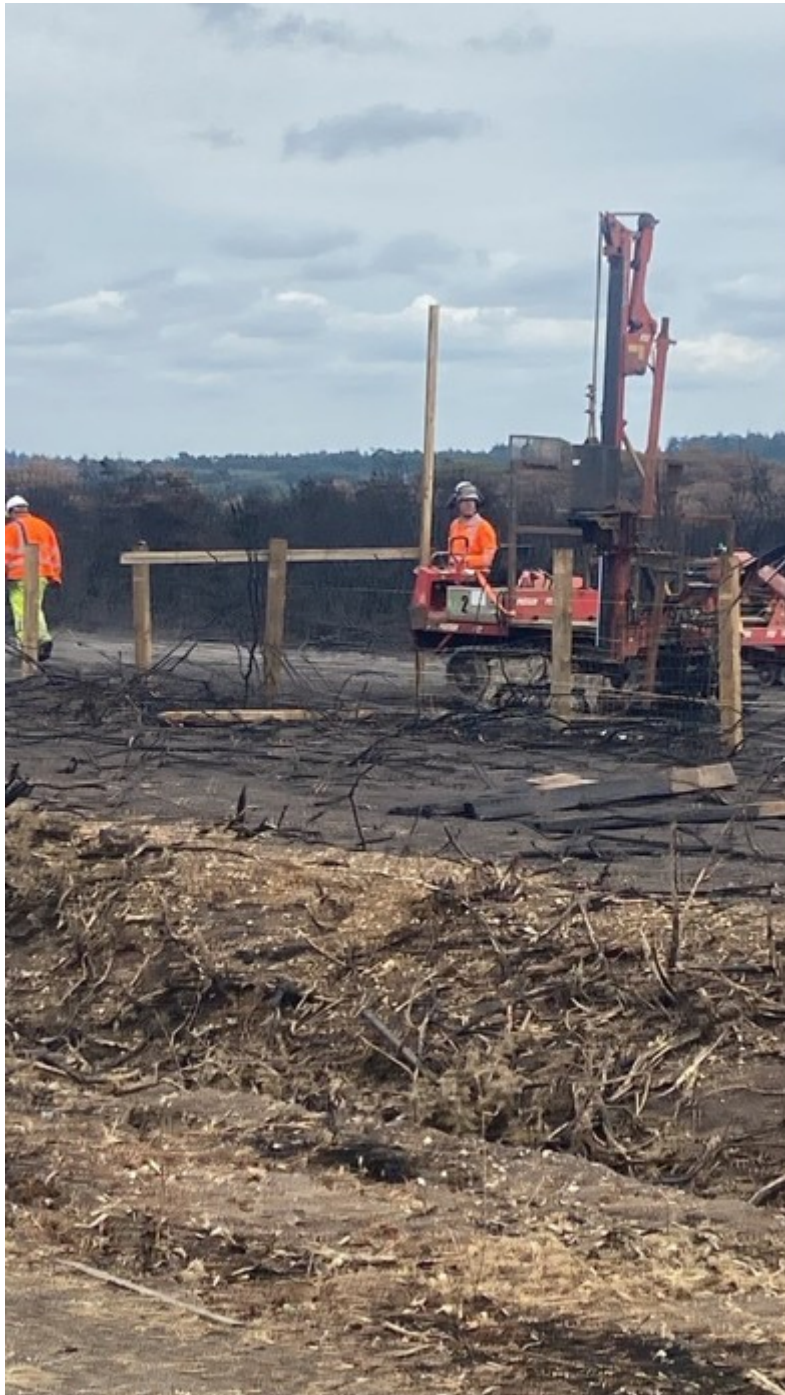
Fencing work taking place.
