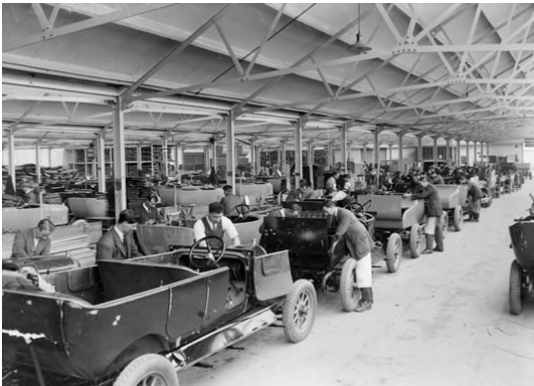
This shot shows the body mounting shop at Morris Motors in Oxford, in 1925
