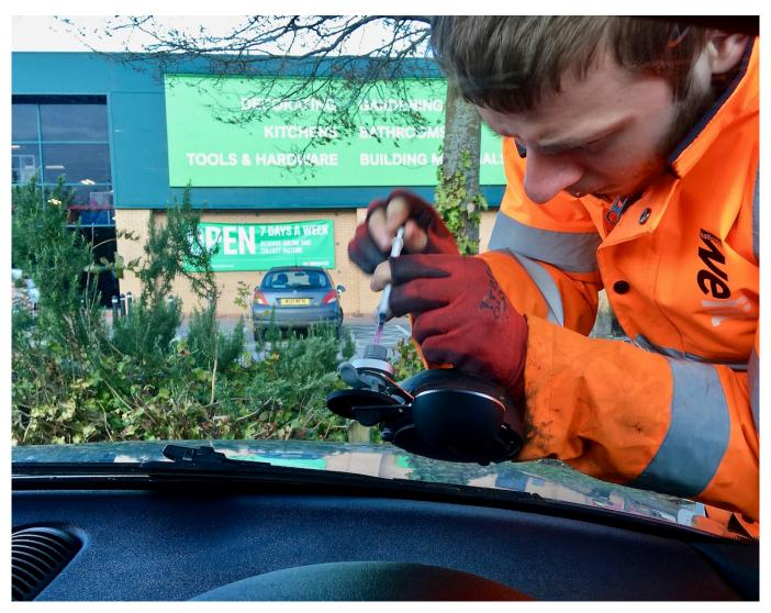
To ensure an MoT pass and to avoid heavy insurance loading on Audi TT windscreen repair, Halfords enacted this one hour repair on star-pattern damage.
